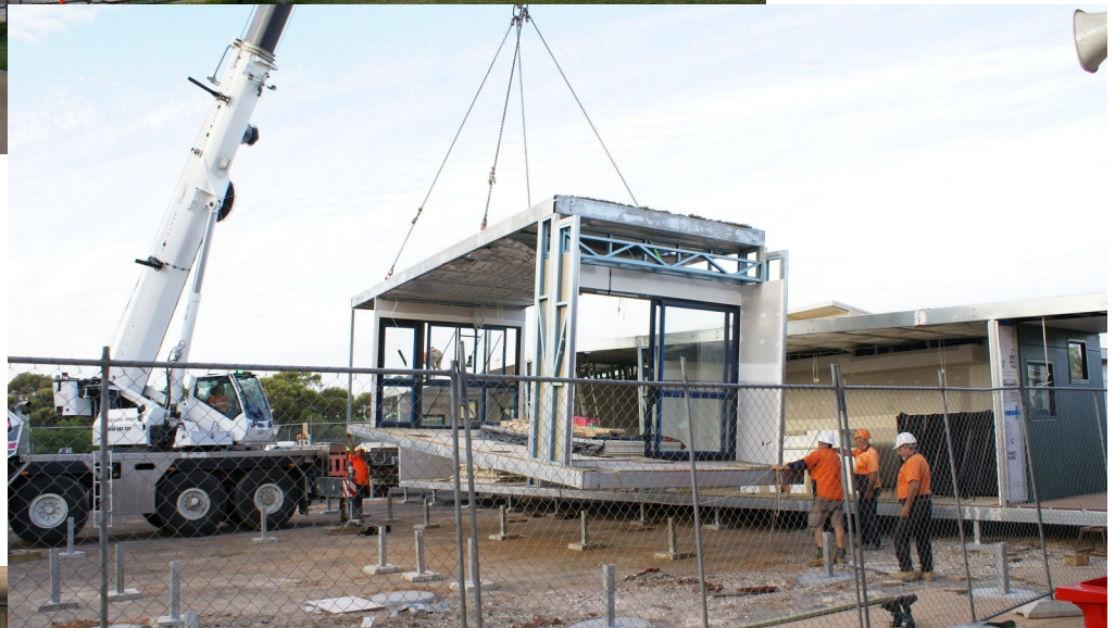
The 8th module being put in place Thursday 22nd Feb.
